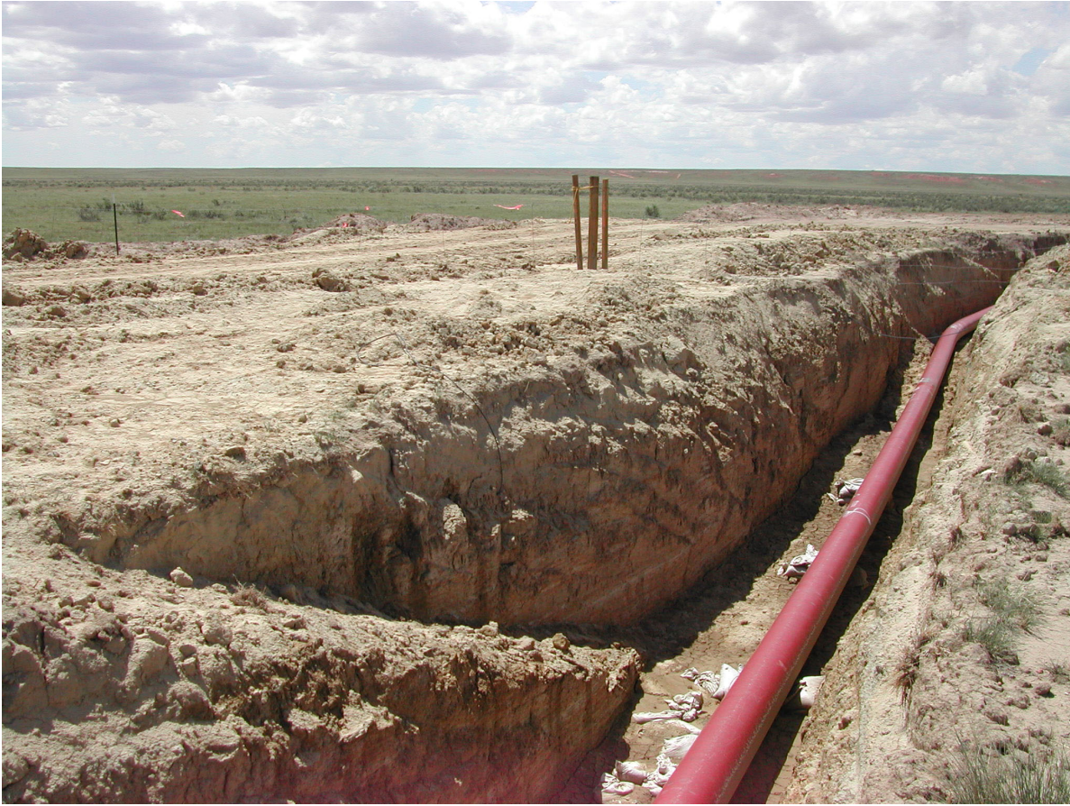
Escape ramps allow trapped wildlife to leave the trench. Photo M. Watson.
