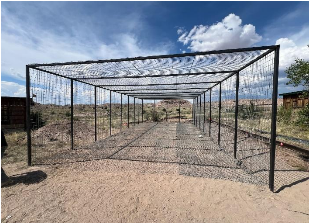
Enclosure Frame and No Dig (July 12, 2025)
