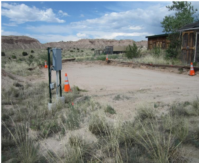
Site Prep (July 1, 2025)
