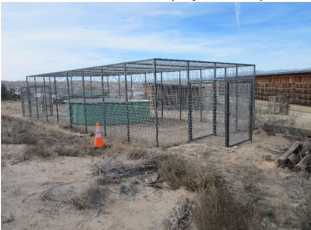
Final Build (December 19, 2025)
