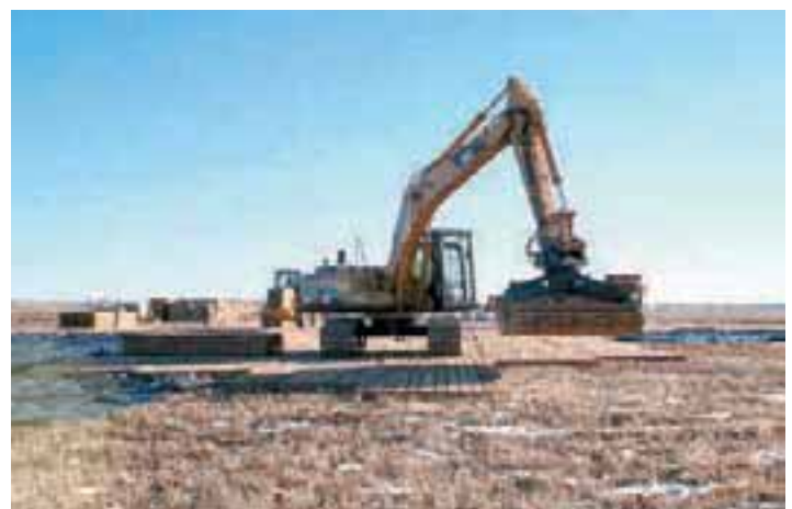
Figure 59. Oak mats being placed directly over drill site to protect top soil. (Photo courtesy of EnCana Oil and Gas).
