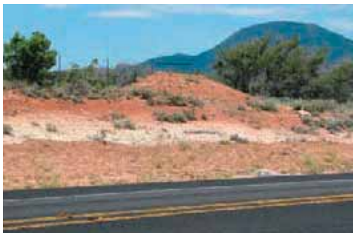
Figure 45. Earthen ramps are often used in the CPE to allow trapped deer and elk to exit roadways protected with high fences. Although high fences are the most effective way to reduce deer-vehicle collisions, they can be very detrimental to migrating deer populations if adequate passage structures are not provided. (Photo by Bruce Watkins/CDOW).
