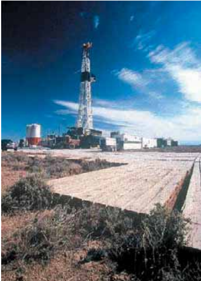
Figure 60. Drilling rig positioned on oak mats. (Photo courtesy of EnCana Oil and Gas).
