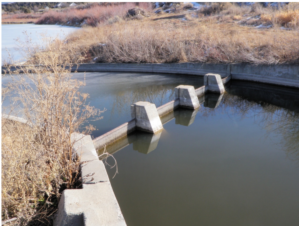
Photo B-9 Fish screen upstream of weir in emergency spillway channel
