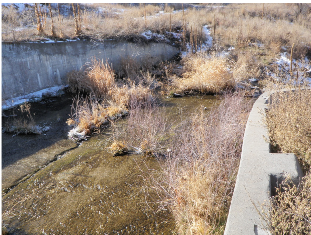
Photo B-10 Chute downstream of emergency spillway weir
