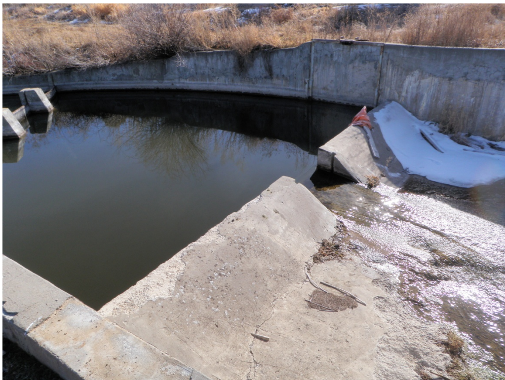
Photo B-8 Emergency spillway weir looking left from dam crest
