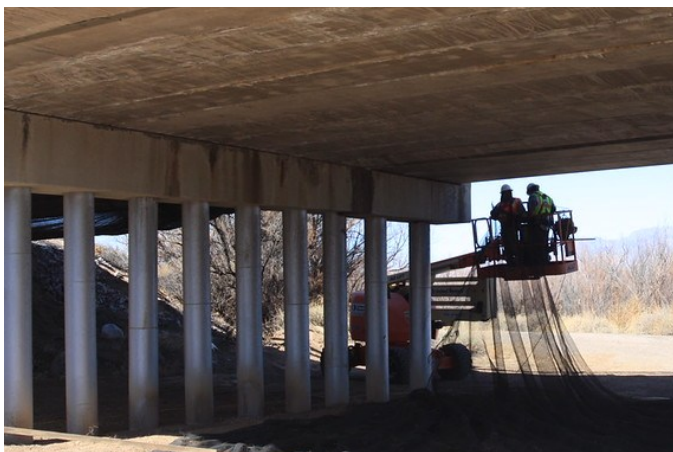
Bat exclusion net installation under bridge. J. N. Stuart.
