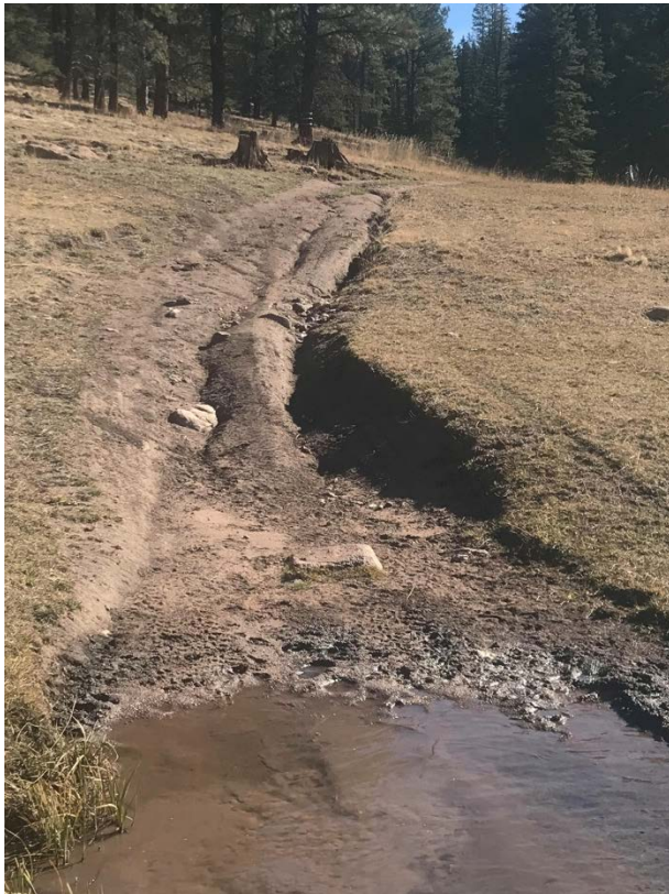
Figure 16. An eroding road crossing contributing sediment into American Creek. Throughout much of the lower reach a non-system user created road parallels the channel.
