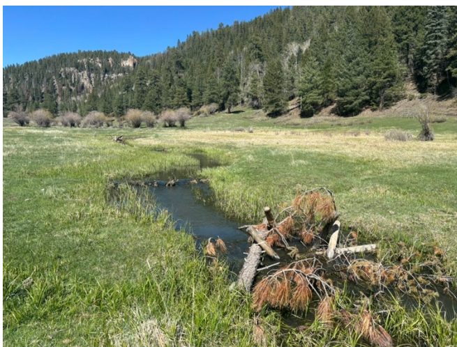
Figure 3. A Post-Assisted Log Structure (PALS) on the Rio Cebolla, Jemez Mountains
