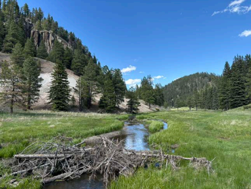
Figure 2. A Large Woody Debris Structure (LWDS) following spring snowmelt floods in 2023. Note extensive racking of small diameter debris. The structure helped to facilitate reconnection of the in-set floodplain.
