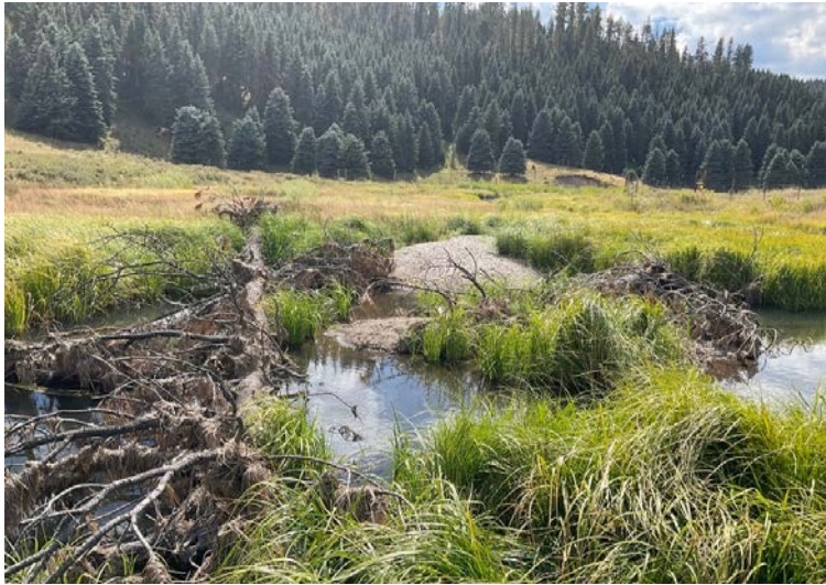
Figure 4. A whole-tree LWDS on San Antonio Creek that caused scour pool development and deposited clean, sorted gravels. Extensive redds were observed at this site.
