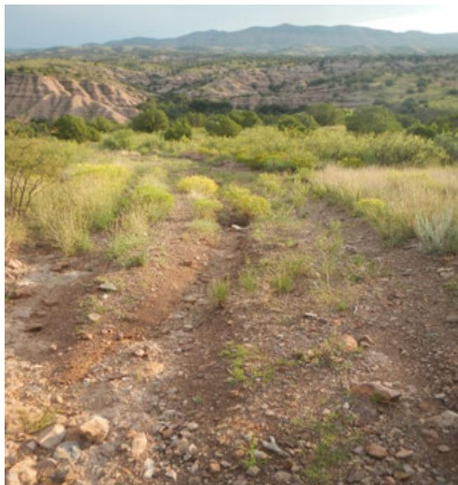
Erosion caused by water entrapment with no turn out. Photo location is South road above gate.
