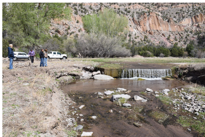
An improperly designed low water crossing on the Tularosa River creates a barrier to aquatic life movement, including the Federally Endangered loach minnow. M. Volke.
