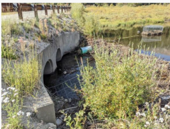
Fence-and-pipe system (photo left and diagram right) with a pipe running from above the obstruction and fencing to the culvert inlet downstream. P. Planer, RangeWorks LLC.
