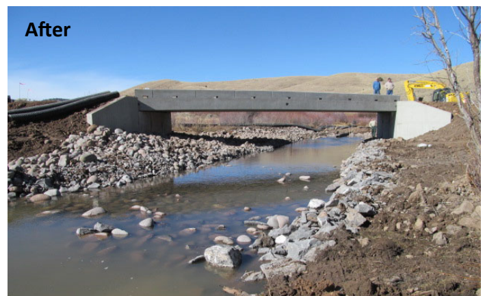
After After: Aquatic life movement is much improved following replacement of the old crossing structure with a bridge. M. Volke.
