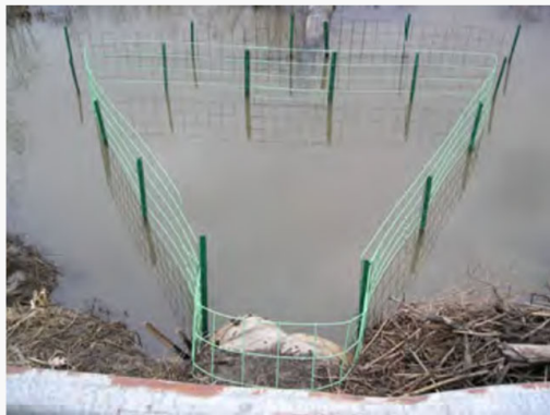
An example of culvert fencing. S. Boyle.
