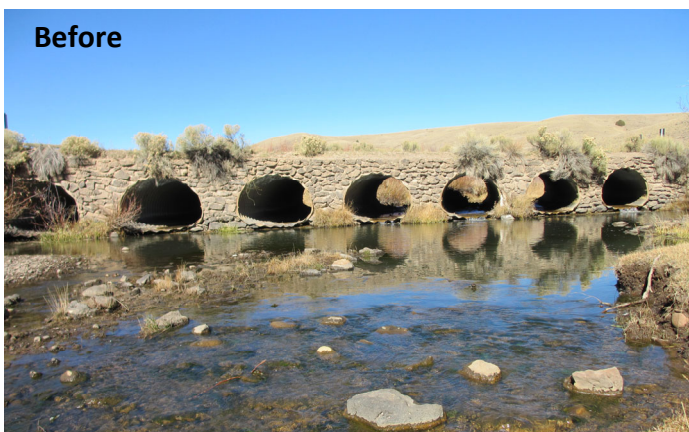
Before Before: A potential barrier to aquatic life movement along the Rio San Antonio on the Carson National Forest. M. Volke.
