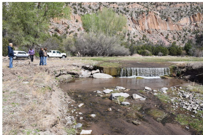
An improperly designed low water crossing on the Tularosa River creates a barrier to aquatic life movement, including the Federally Endangered loach minnow. M. Volke.
