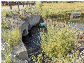
Fence-and-pipe system (photo left and diagram right) with a pipe running from above the obstruction and fencing to the culvert inlet downstream. P. Planer, RangeWorks LLC .
