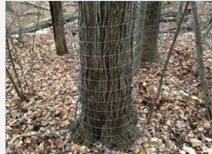
Protective fencing around a tree. CDOT
