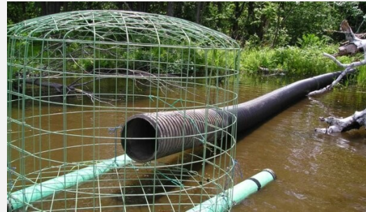
A pond-leveler being floated into place prior to submersion. The Beaver Institute
