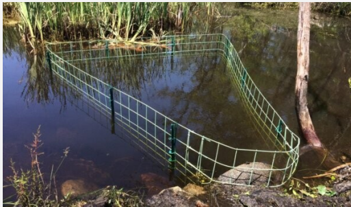
Culvert protective fencing. The Beaver Institute
