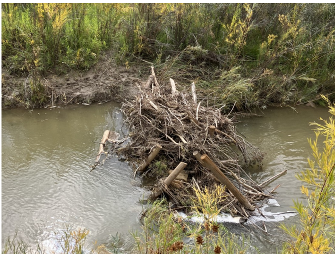
Post-assisted Log Structure (PALS) near Mancos, Colorado. J. Marchetti
