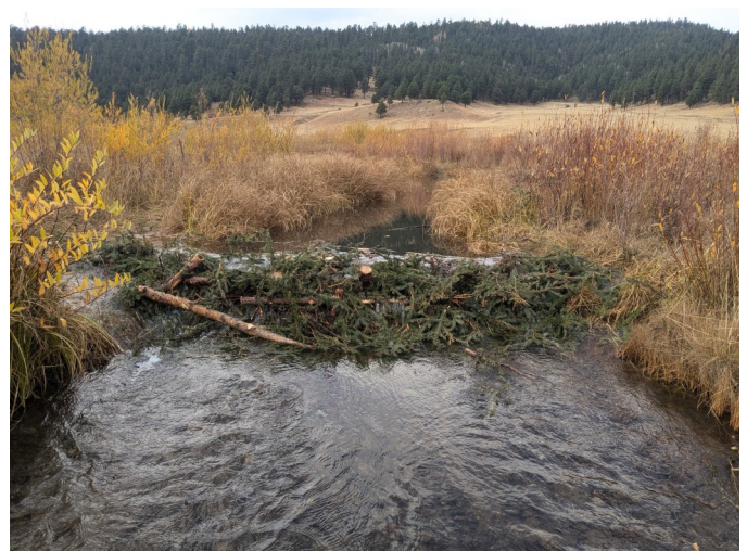
Beaver dam analog (BDA) constructed on San Antonio Creek in Valles Caldera National Preserve, NM. P. Watson
