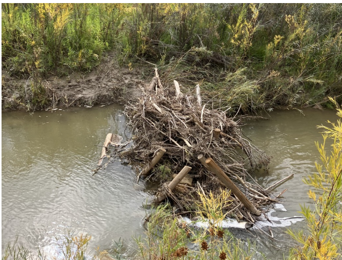
Post-assisted Log Structure (PALS) near Mancos, Colorado. J. Marchetti
