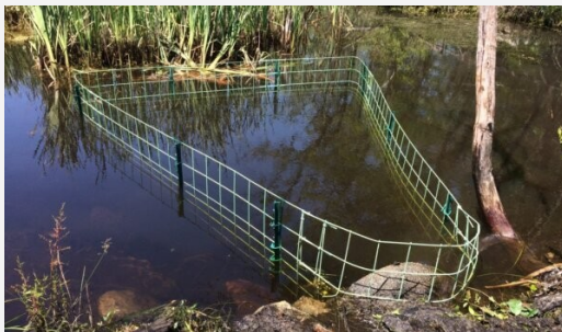
Culvert protective fencing. The Beaver Institute
