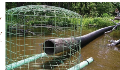
A pond-leveler being floated into place prior to submersion. TBI
