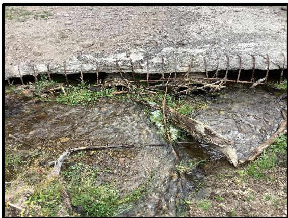
Figure 1 Culvert number 115 on the Rio Cebolla (Photo credit: Cascade Conservation)
