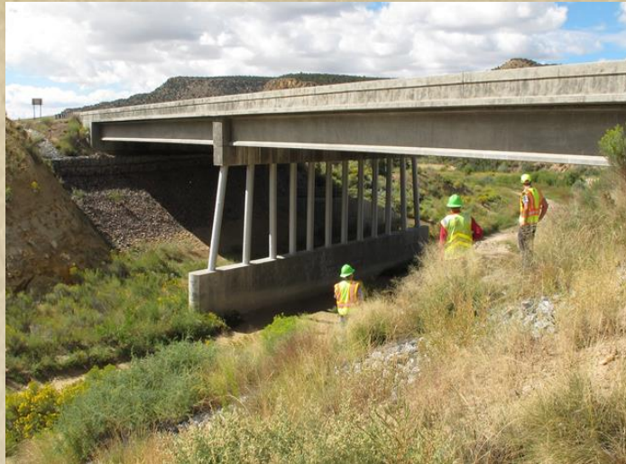
U.S. 550 bridge over Rio Puerco south of Cuba
